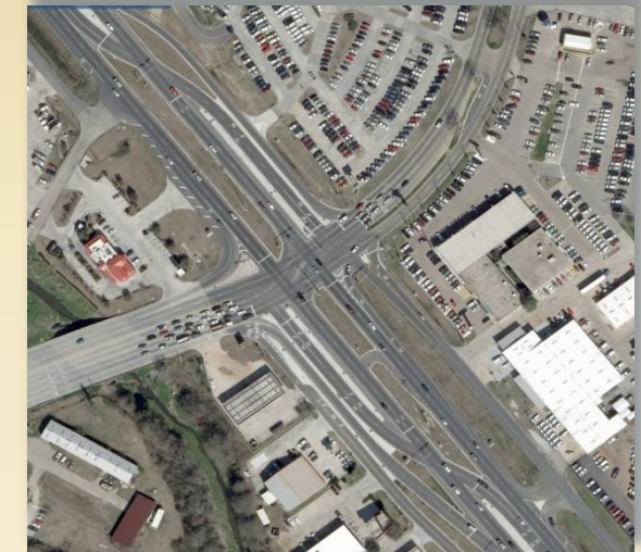
Two-Leg CFI at Siegen Lane & US61/Airline Highway in Baton Rouge, LA (Source: Google Maps, 2008)
